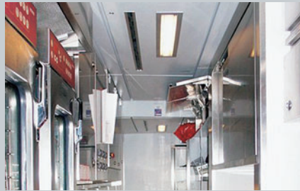
Linear air diffuser type LDB 20/8/1
